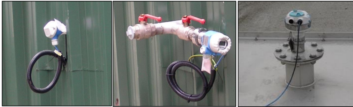
Picture 2: Measurement devices for temperature and level sensors (right: ultrasonic measures from top).
