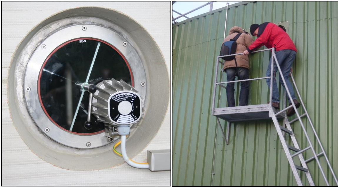
Picture 7: left: inspection hole with camera system, right: manual inspection.
