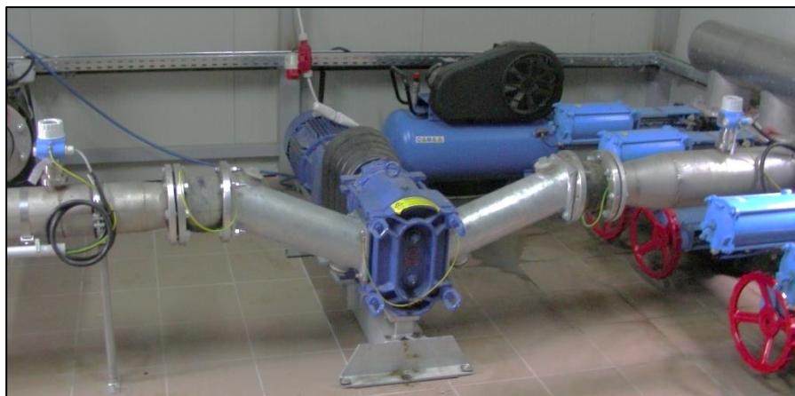
Picture 3: Pumping station with pressure sensor before and after the pump to detect distortions.
